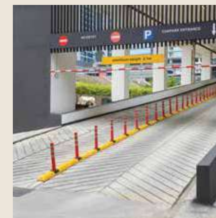
Express car park ramp to multi-level parking
